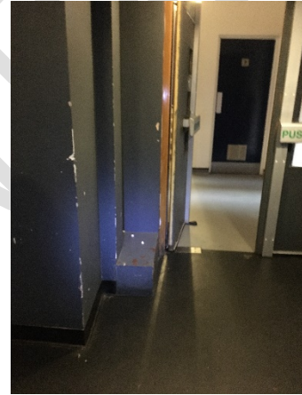
Nightclub area: SU staff aware of custom and practice to wedge open fire doors. Daily check needed, removal of wedge, and discussion with cleaners.
