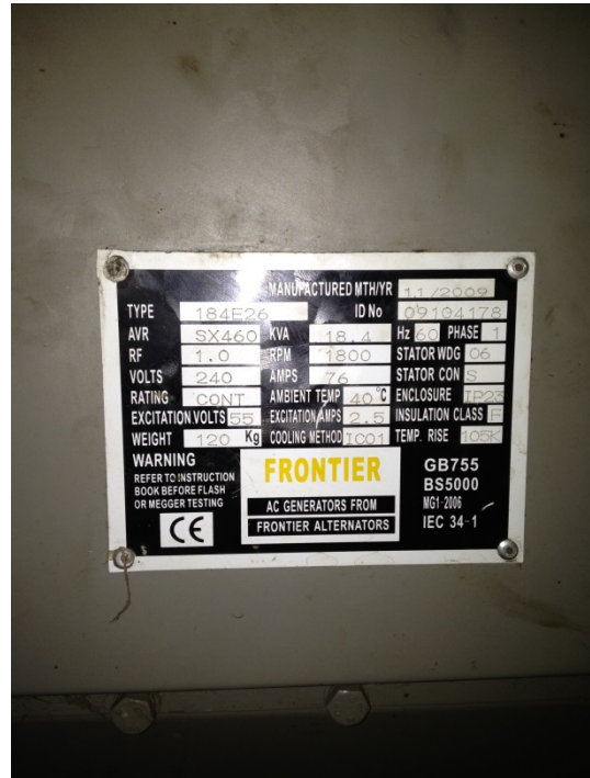
Alternator Specification (Alternator is belt driven)
