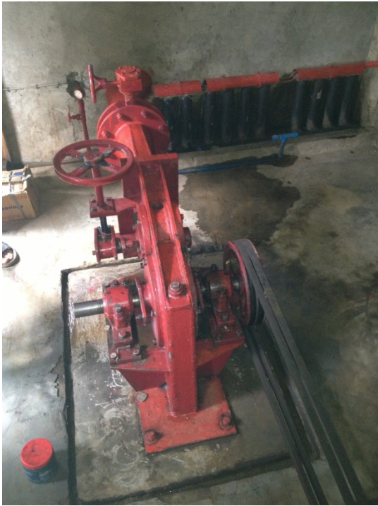
Micro Hydro Power Plant (Turbine)
