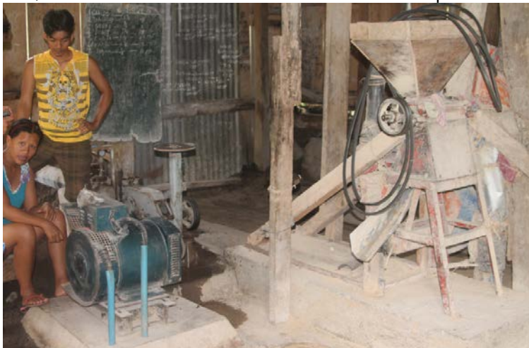
MHP powerhouse in Buneg (turbine, alternator and rice mill)
