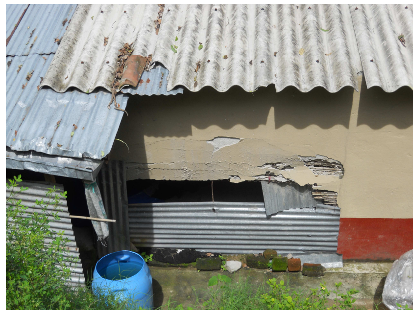
Wall destroyed by a landslide in Costa Rica
