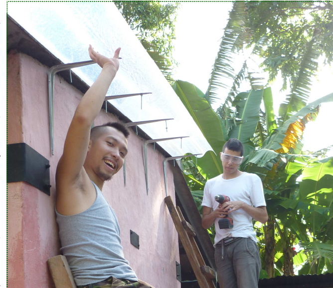
Installing the roof extensions in 2011
