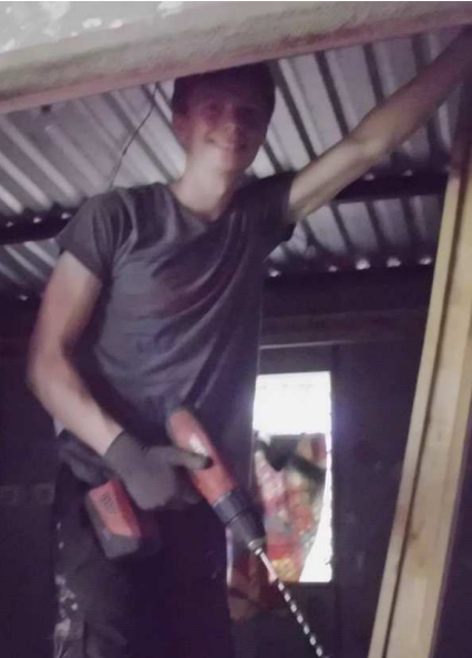
A student drilling holes
