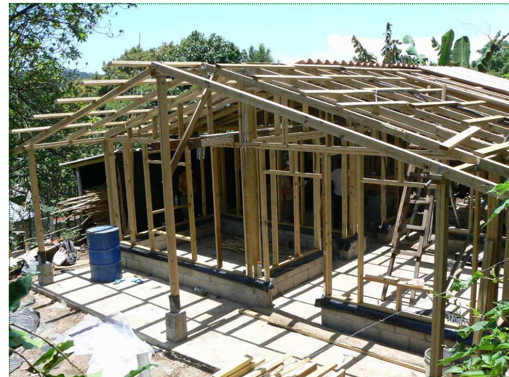
Prototype house from the 2012 project during construction
