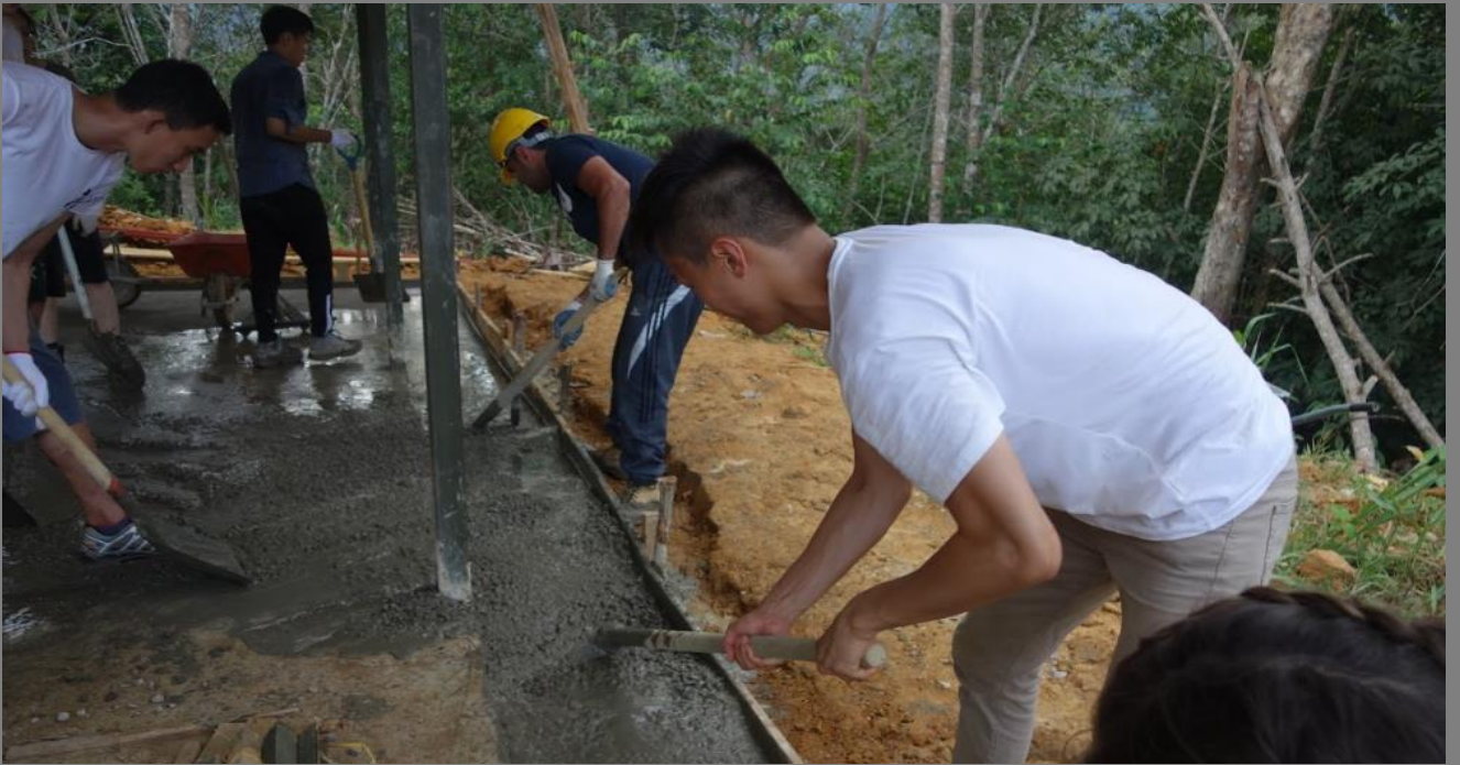
Figure 28: Casting of the outerslab.
