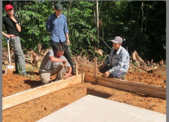
Figure 20 Setting out.
