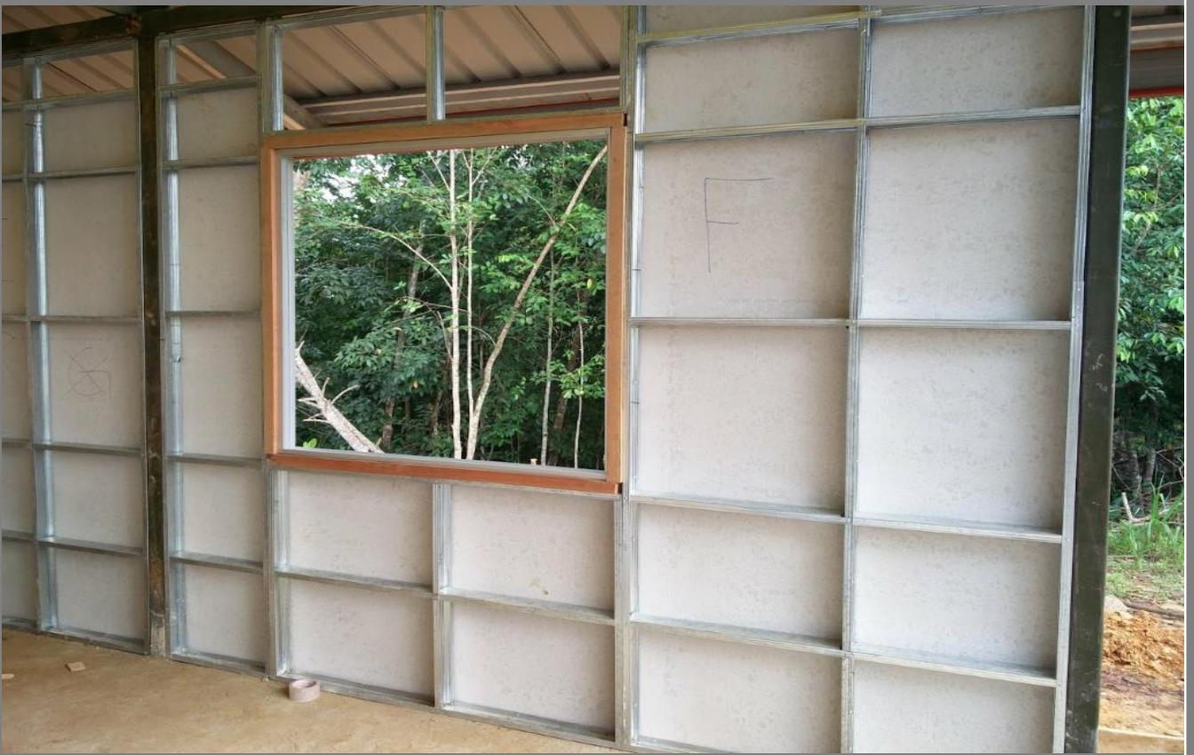
Figure 31: Wall panels attached onto the wall studs.
