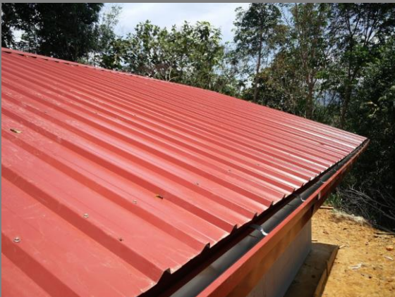
Figure 30: Gutter and fascia.
