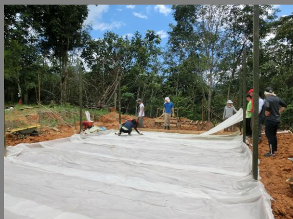
Figure 27: Concrete slab water proofing.
