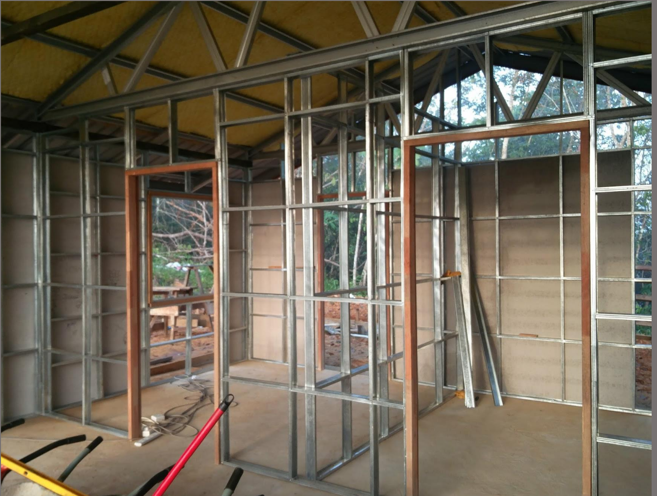
Figure 13: Internal wall frames of the kindergarten.
