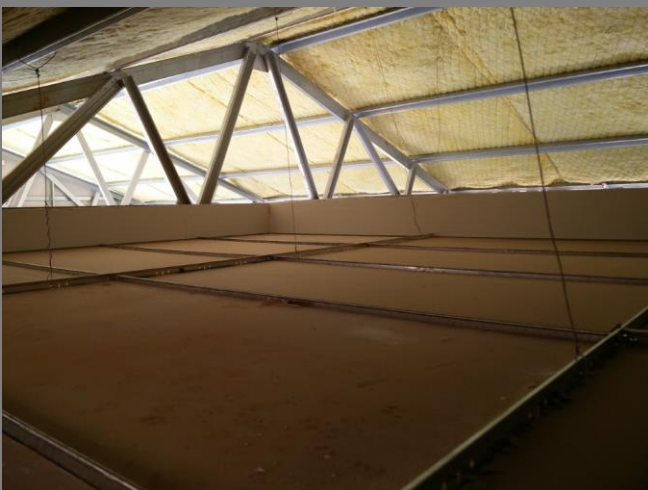
Figure 38: Ceilings suspended from the battens
