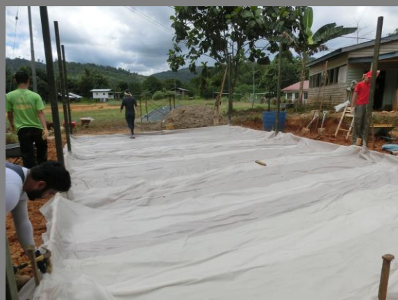
Figure 26: Polyethylene sheets positioning.
