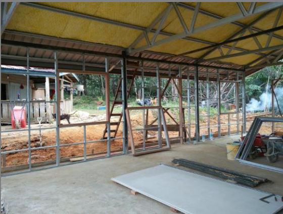
Figure 29: Wall studs.
