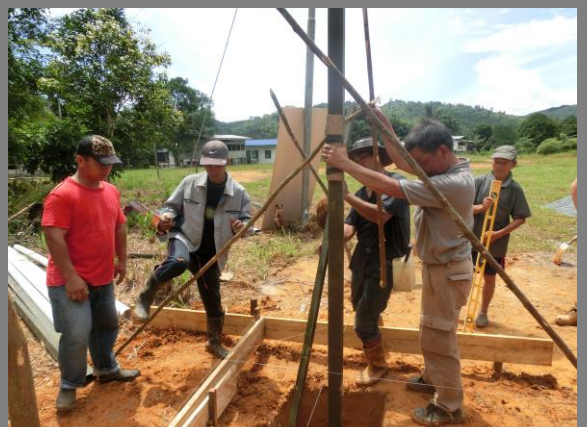
Figure 21: Column propping
