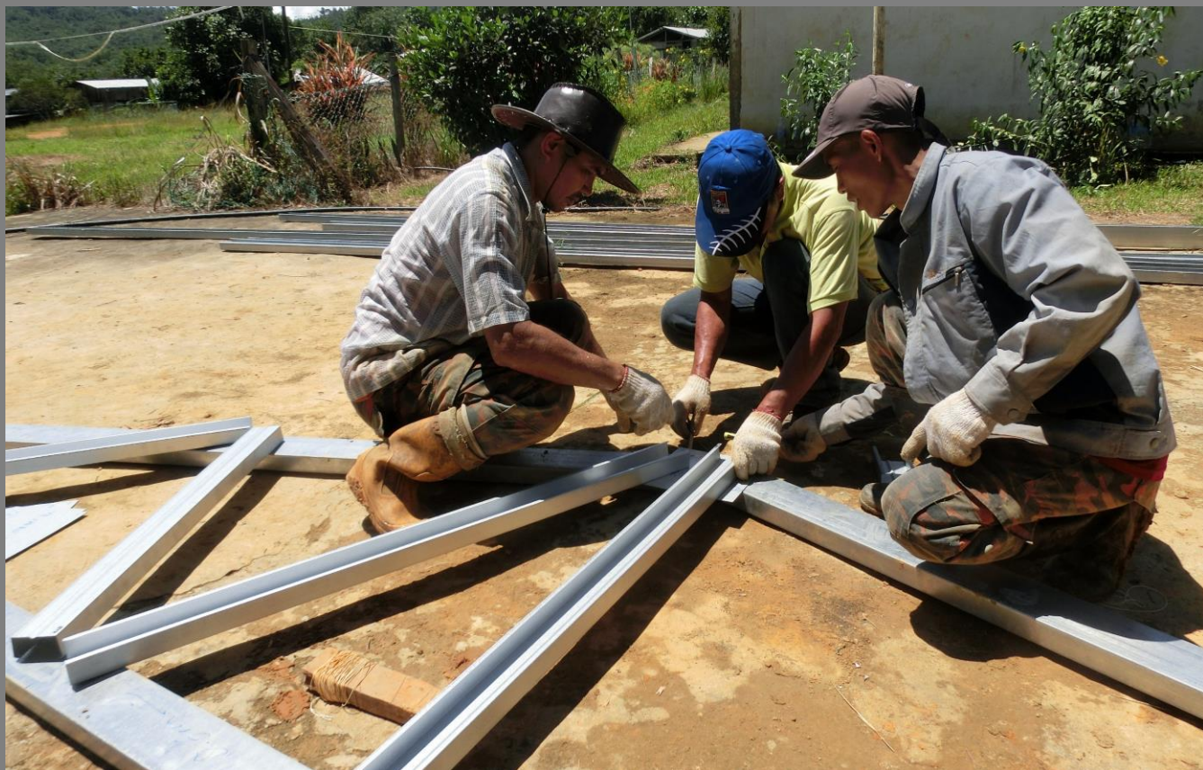
Figure 25: Truss assembly.
