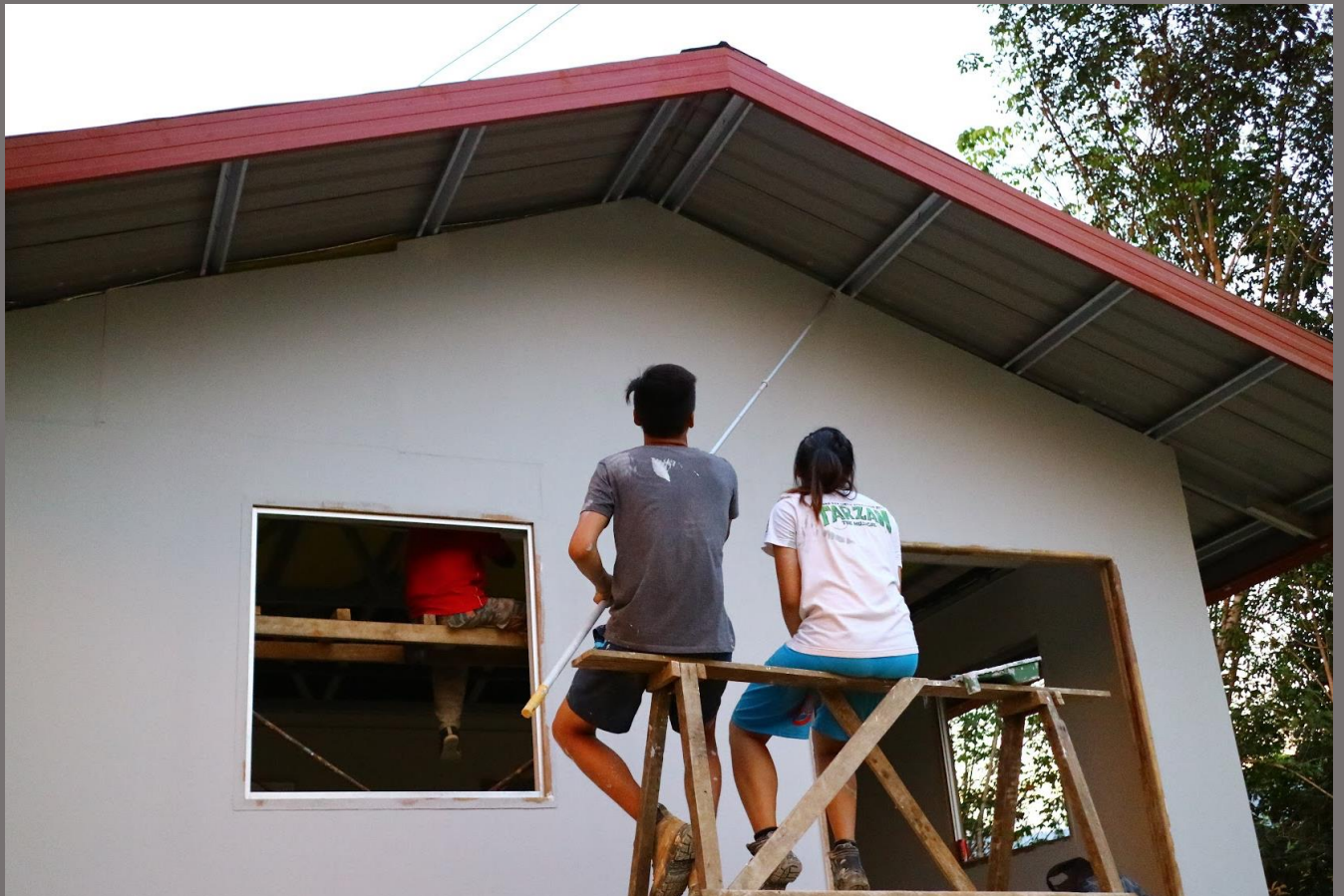
Figure 14: Jeffrey and Shi Jinn painting the prefabricated cement wall panels.
