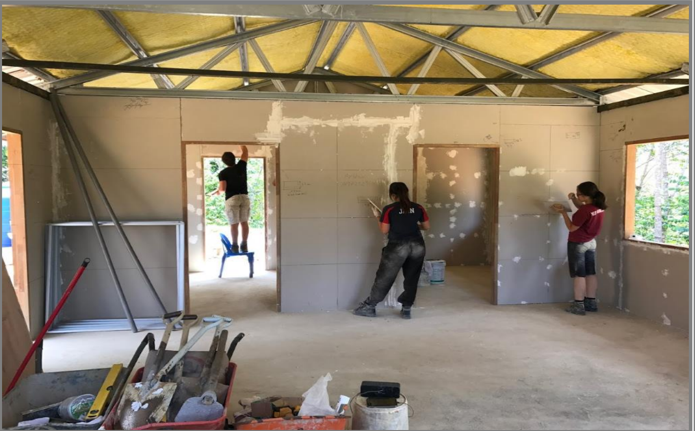
Figure 37: Plastering the wall panels.
