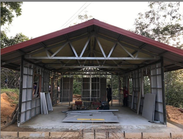
Figure 32: Wall studs overview.
