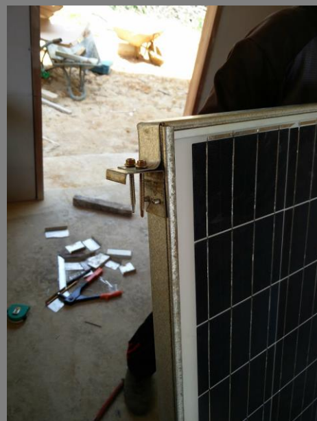
Figure 36: Housing lock.
