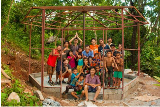
FOUNDATION AND FRAME BOTH IN PLACE
